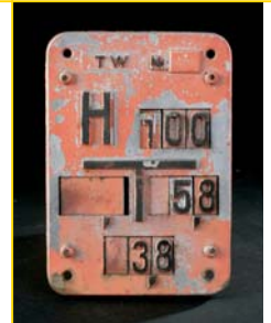
Signs show the size of water pipes and position of hydrants.
